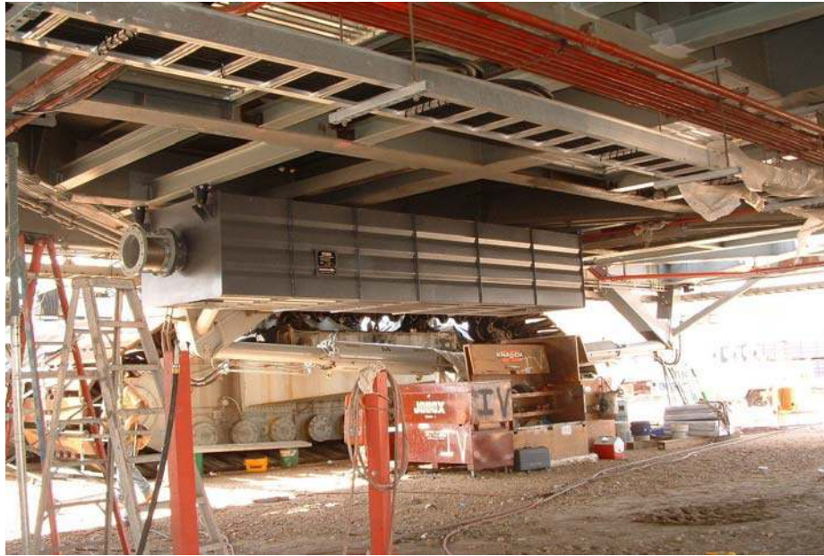
Figure 2: One of two New ALCO Engine Mufflers (White Engines have only 1 Muffler)
