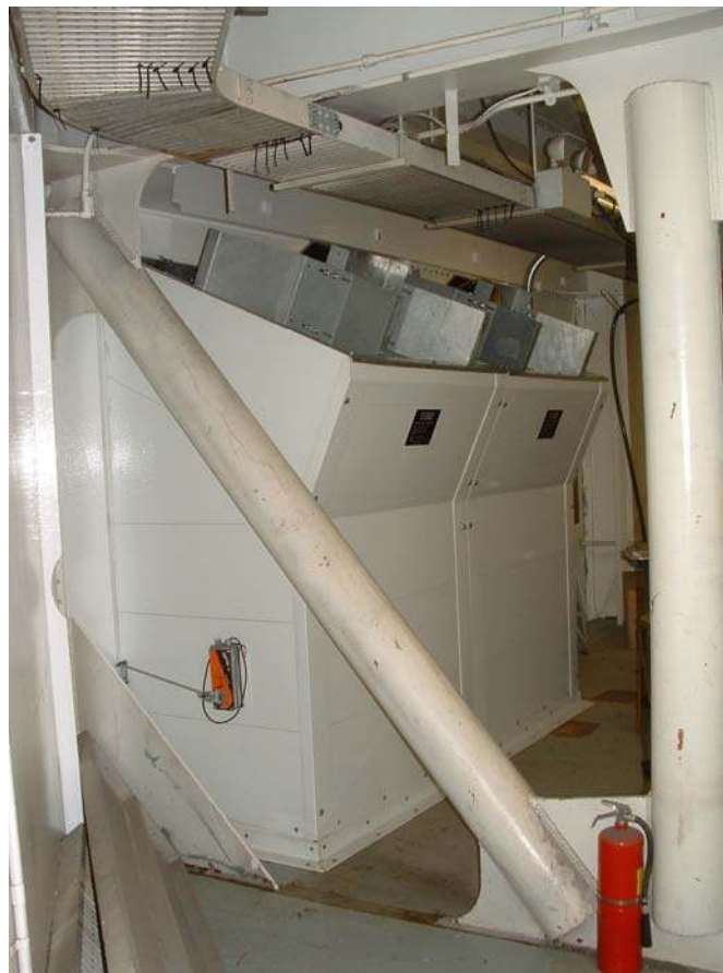
Figure 6: New double Exhaust Hoods installed in place of Old Inlet fans
